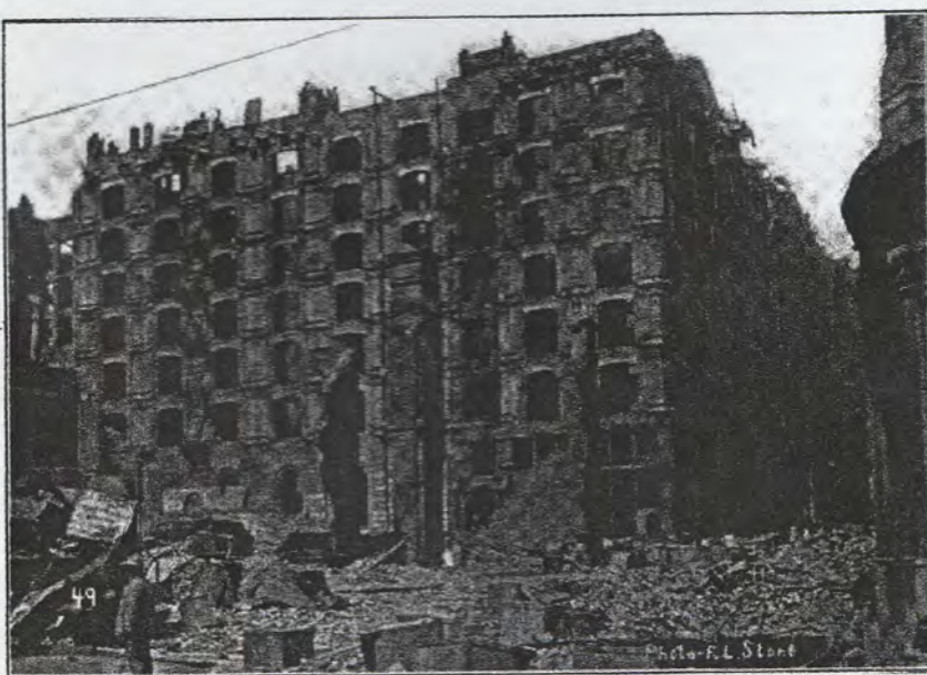
THE PALACE HOTEL. Northwest Corner of Market and New Montgomery Streets. The exterior walls are of brick, well tied by steel rods and bands. The interior dividing walls or partitions are also of brick. The floors and interior finish were of wood. The excellent design and workmanship of the walls prevented any material damage by the earthquake. Fire consumed the wood floors and all the combustible contents, leaving only the walls, which remain in good condition. It is the best preserved building of the non-fire-proof type in the burned district.
